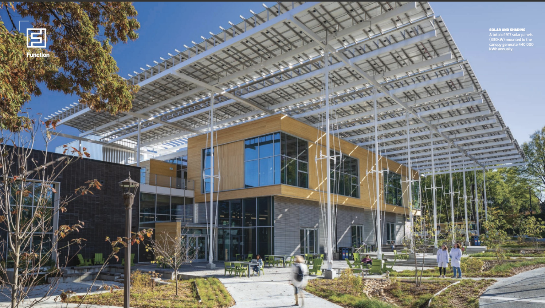
The Kendeda Building's canopy shades the building to reduce cooling demand, generates electricity via solar panels, collects rainwater, and is also a defining architectural feature.
